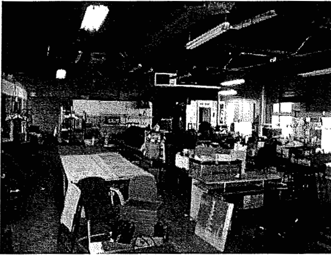
VIEW OF THE FIRST FLOOR OF THE 2-STORY BUILDING (GARAGE SPACE)
