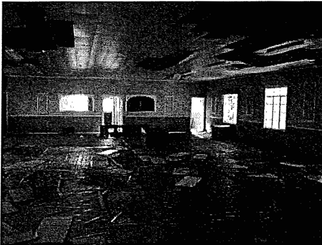
VIEW OF THE SECOND FLOOR OF THE 2-STORY BUILDING LOOKING TOWARD THE KITCHEN AND RESTROOMS
